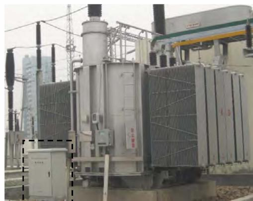
Fig.7 Test installation schemes of oil chromatographic
